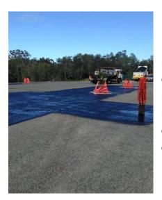
Road construction includes boxing out, proof rolling, removal of soft spots, installation of subsoil drainage, and importing of quarried road base materials. Compaction and testing, to achieve required finish levels including final trim for the options of concreting, asphalt or 2 coat seal for commercial and residential projects.
