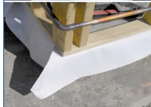
**HomeGuard DPC** (Damp Proof Course) is a tough 500 micron UV stabilised polymer sheeting containing Biflex Termiticide that offers both perimeter subterranean termite protection and damp proofing through the one installation.
