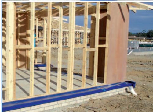
**HomeGuard Blue** is manufactured in Australia from 300 micron, UV stabilized blue polymer sheeting containing Biflex Termiticide which provides perimeter subterranean termite protection. This material is not rated to provide a moisture proof membrane.
