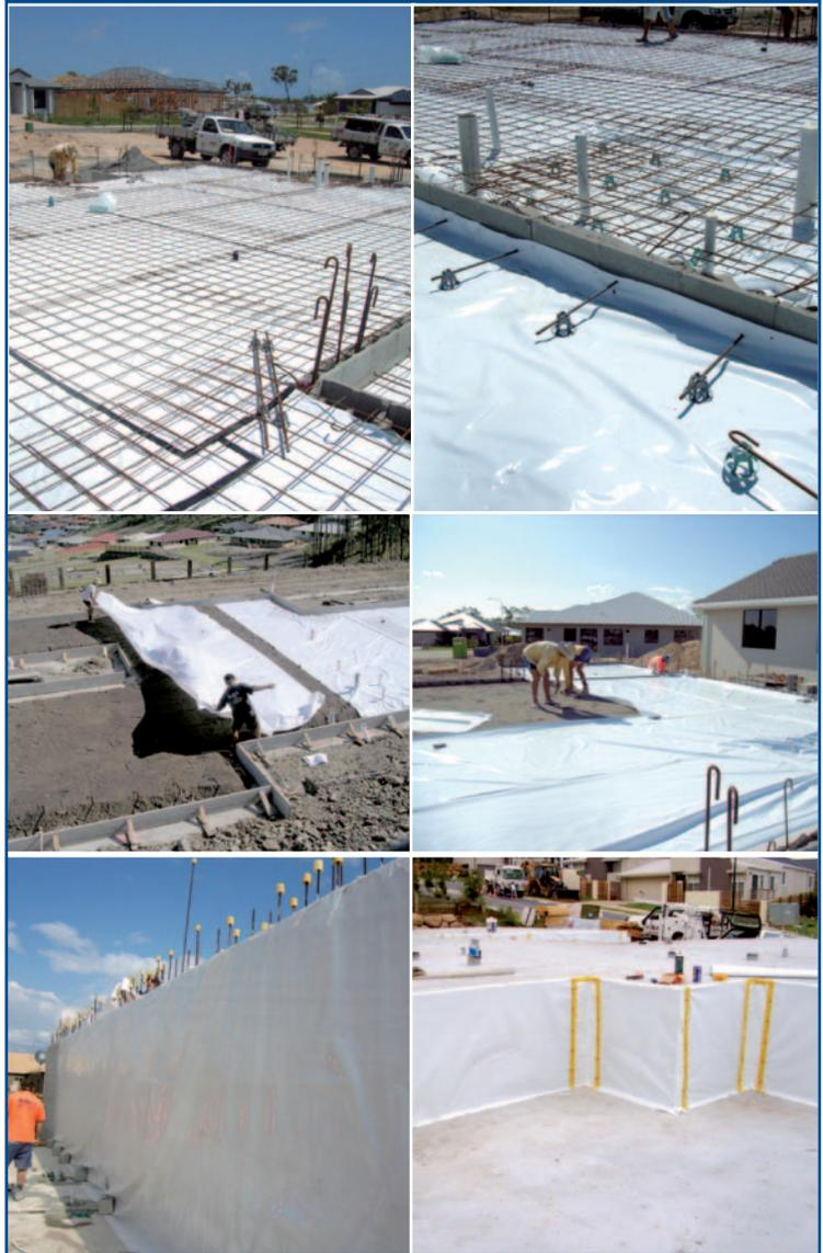
**HomeGuard TMB** (Termite & Moisture Barrier) as the name implies offers the builder both a moisture barrier and a subterranean termite barrier in the one installation. TMB is available in a 4m x 50m sheet.
