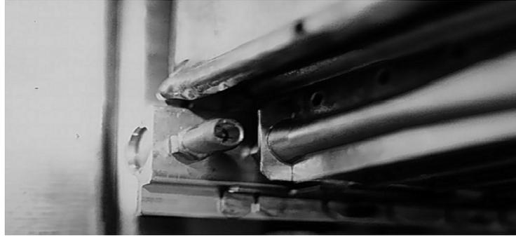
8. Minimum Gas Pressure Adjustment. Attach manometer to burner test point (see picture above) Set water flow selector fully clockwise (hot position). Move gas slide to left side, single flame symbol, open hot tap fully. Turn adjustment screw (Position C in picture below) located on left hand side of gas valve at a 45° angle to correct pressure. Anti clockwise to decrease minimum burner pressure.
