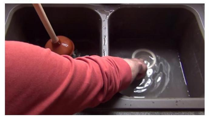
Toilet discharge pipes can get blocked when you put the wrong things down the toilet, such as sanitary pads, food scraps, rags, cans, bottles, paper, fat and grease. Similarly, waste water pipes from basins, sinks, and laundry tubs can also be clogged by food waste, tea leaves, grease, lints, hair and other rubbish.
