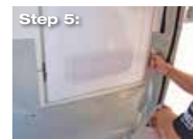
Step 5: Install draft skirt
