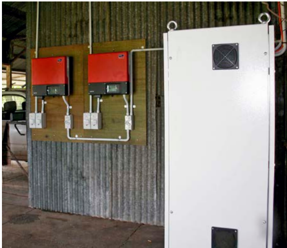
↑ The two SMA grid-interactive inverters at left, with the battery and equipment enclosure at right
