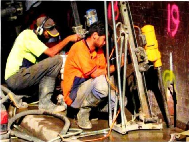
The project required the drilling of 22 x 175mm $\emptyset$  holes at angles of 11° and 13° up to 4 metres deep into each of the two massive brick and concrete abutment structures as preparation for grout stabilisation injection. This was made necessary by the increased loads associated with the replacement of the 1930s era riveted steel bridge beams with a precast & prestressed concrete deck.
