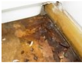
Identify wet rot - rotten floor
