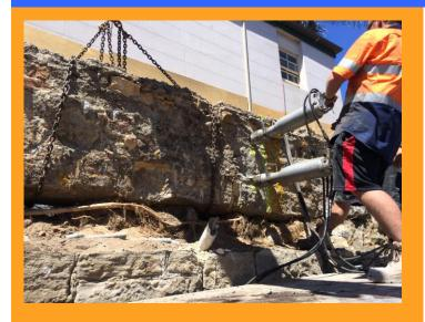
We looked at wire sawing it into blocks but because it was adjacent to a footpath thought it would be safer to use the Darda splitters.
