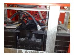
FPA Australia is aware that reported failures or ruptures are likely to be the result of incorrect charging of flooded-cell lead-acid automotive batteries that have been poorly maintained. Incorrect charging can cause electrolysis of the electrolyte fluid (sulphuric acid and water) that surrounds the lead plates within the battery. Electrolysis produces hydrogen and oxygen gases and depletes the electrolyte of water. Whilst these types of batteries typically have vent holes to allow gases to
