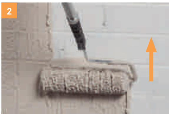
Stir contents of *Dulux Texture Full Cover Roll On* with a broad flat paddle using an up and down scooping motion. Pour contents into a deep roller bucket or tray. Using a *Full Cover Texture Roller*, load the roller, then deliver material to the wall in vertical strips to ½ to ¾ metre from the ground upwards with a smooth steady action. Avoid rolling downwards as excess material may fall from the roller. After 4-5 roller widths have been applied the levelling process should be commenced.
