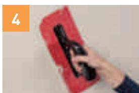
Finishing must continue before the skin dries. Finish (float) the levelled area in circular strokes to further fill and even out material. Use harder pressure to fill low spots. Work in larger, lighter strokes as material levels out. Use a clean bucket of water and a sponge to clean and keep the plastic float moist.
