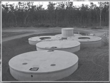
We will build inground tanks with roof loading from non-trafficable to capable of carrying a semi trailer. Up to 2 metres fill over roof.
