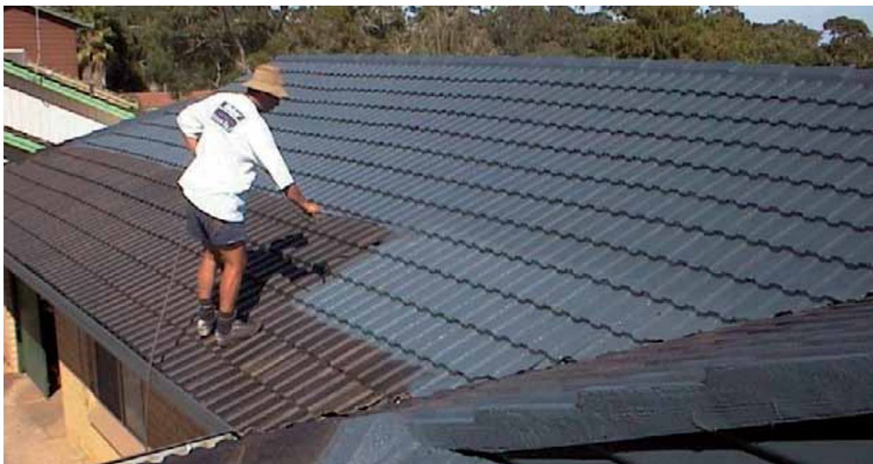
Applying first coat Next Generation Roof Membrane
