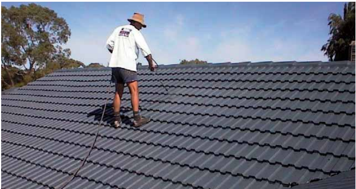
Applying second topcoat Next Generation Roof Membrane
