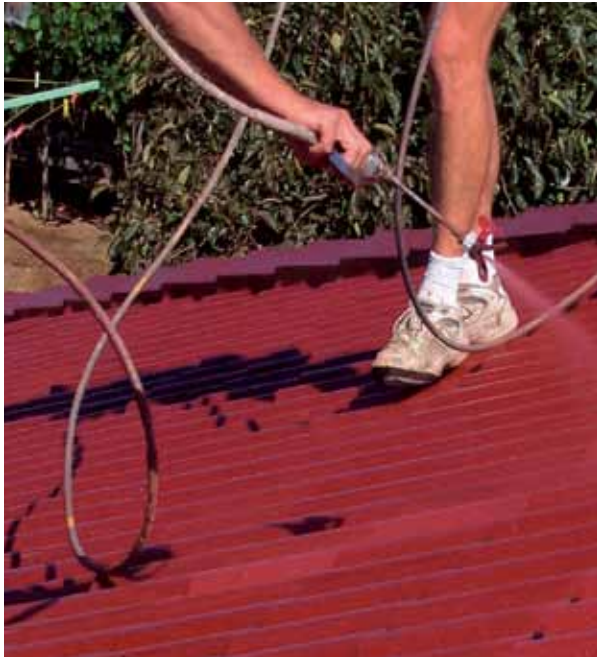
Applying second topcoat Next Generation Roof Membrane
