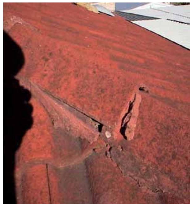
Failed pointing & bedding
