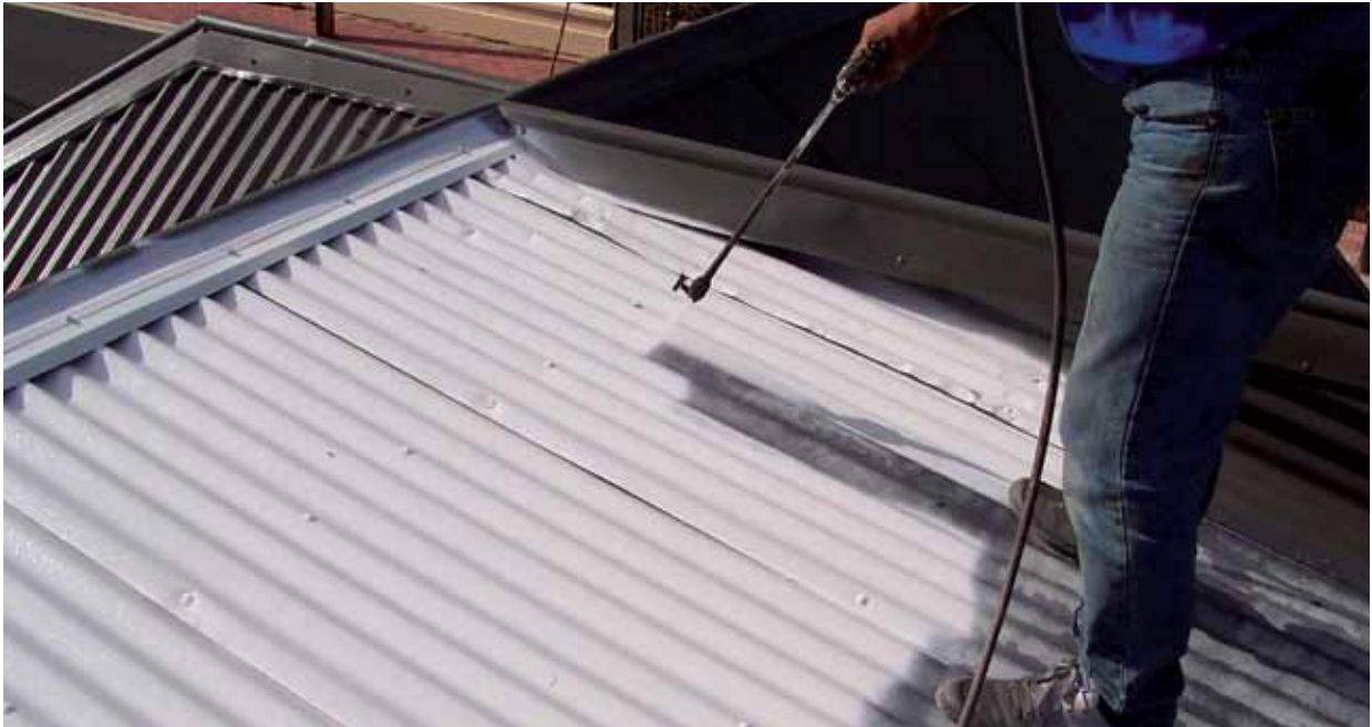
Applying Cool Roof
