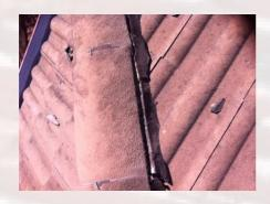
2. Check for <u>broken ridge and gable</u> <u>tiles</u>, which may cause leaks
