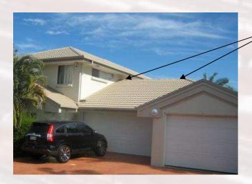
3. <u>Condition of ridge capping</u>. E.g. condition of bedding and pointing. Major or minor cracks in the bedding and pointing can cause leaks or dislodgement of the ridge.
