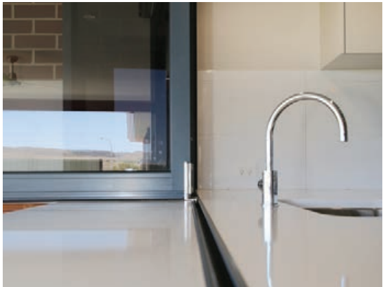
Flush Bi-Fold window sill for smooth transition in kitchen servery application.
