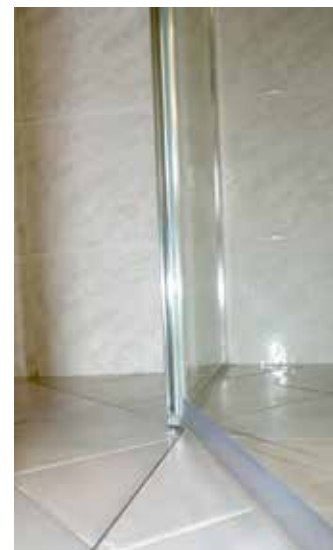
Fitted inside recessed floor.
