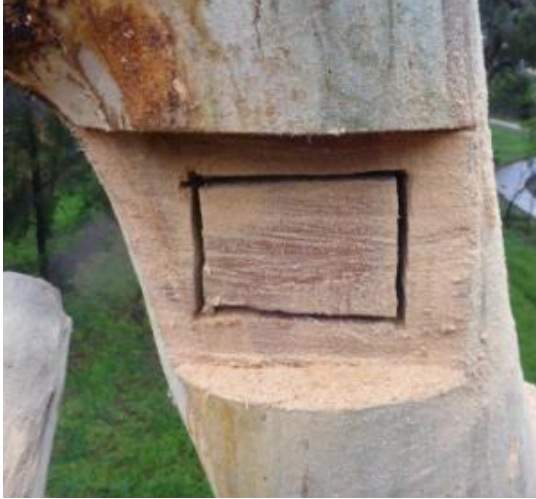
Figure 7: Cavity boring cuts
