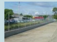
Perimeter Security Fencing
