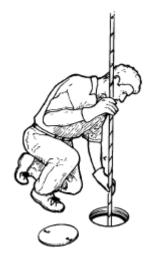
3) Withdraw it completely, noticing the size and position of the scum mark and the depth of the sludge.
