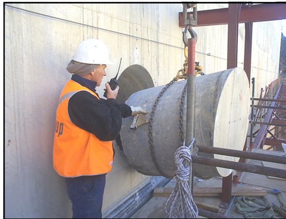
Core holes at Warragamba dam 950mm diameter x 1100mm deep
