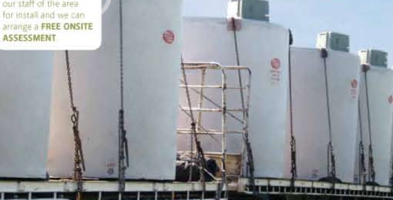
A typical installation of a 10,200L squat tank below a turf area. These tanks are ideal for high water table or rocky areas with difficult excavation.
