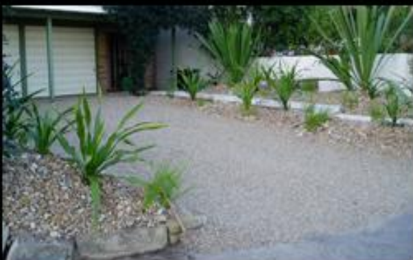
Nepean River Gravel Two Coat Seal Driveway
