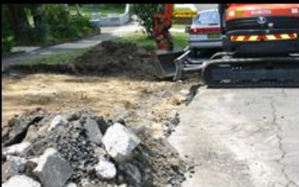
Excavation of Roadway
