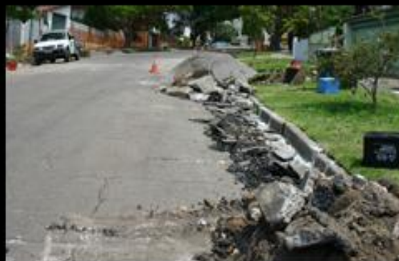
Excavation of Roadway
