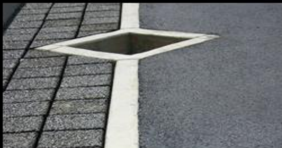
Asphalt with Concrete Kerb and Eco Paver Edge
