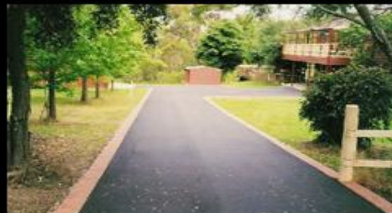
Asphalt Driveway with Paver Edge
