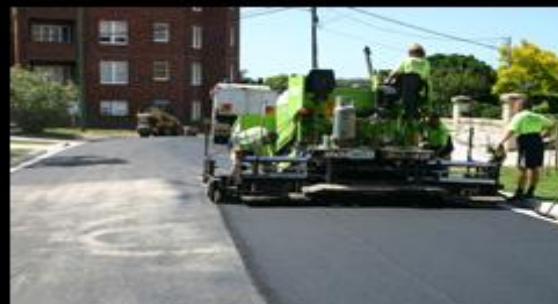
Machine Laid Asphalt Roadway in Progress
