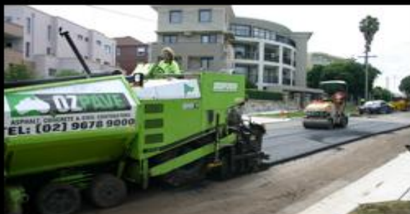
Machine Laid Asphalt Roadway in Progress
