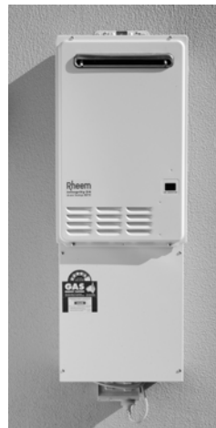
Fig 4.3: Rheem Integrity recess box and pipe cover
