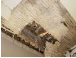
Identify Dry Rot brittle wood
