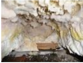
Identify Dry Rot cotton wool like sheet
