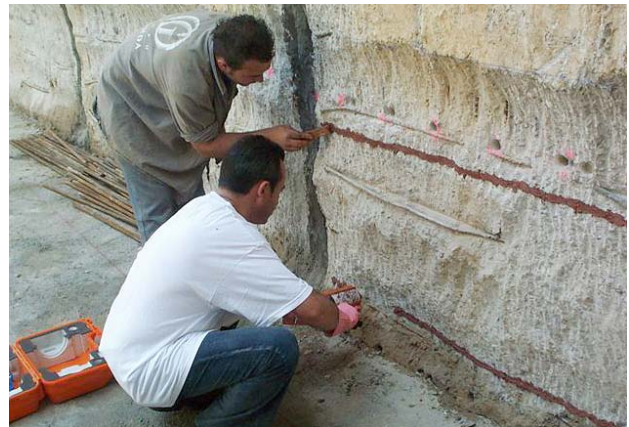
Connection diaphragm walls
