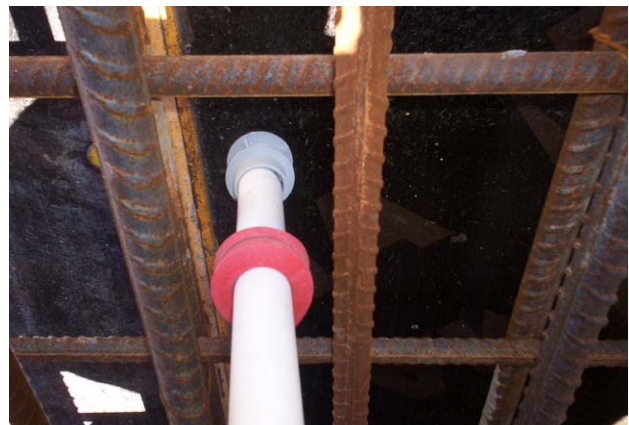
Formwork spacers
