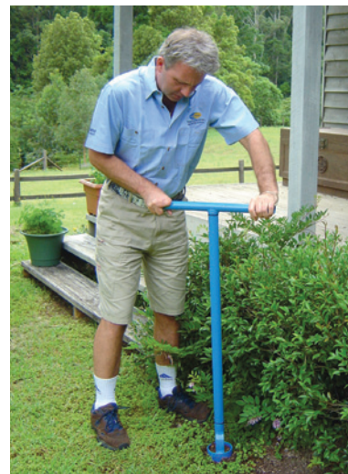
Using auger to place Exterra Station.
