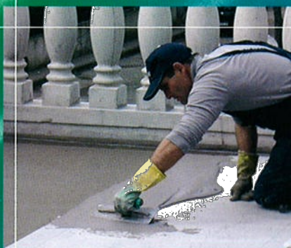
Application by trowel
