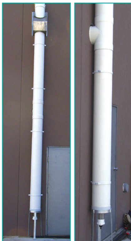
► 225mm Commercial Downpipe First Flush Water Diverter. The T-junction is installed connecting to the rainwater tank located inside the building.
